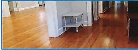
Completion of floor restoration
