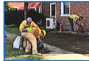
8/27/20 gas connection completed
