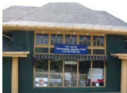
Phillipsburg Union Railroad Station
