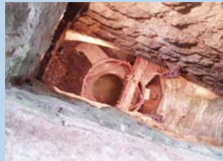
View looking down at underground equipment
