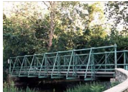
Pony Pratt Truss Bridge Copyright P.S. Green
