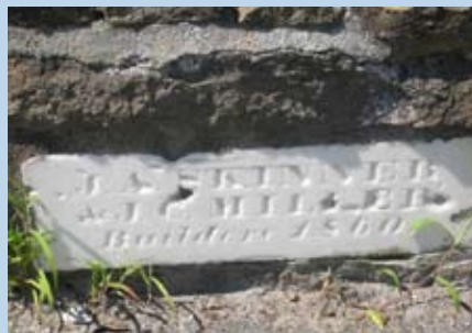
1860 Stone Arch Bridge and Builder's Plaque at Miller Farmstead
