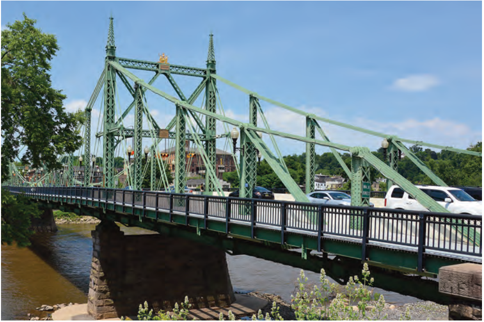
Northampton Free Bridge. Phillipsburg, NJ and Easton, PA.
