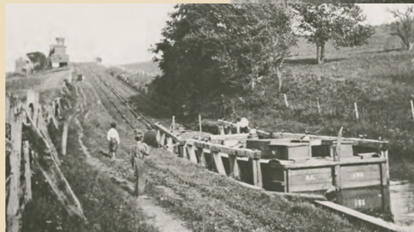
At Inclined Plane 9 West, canal boats were floated onto a cradle car and pulled, by water power, 100 feet up the plane to the next level of the canal.
