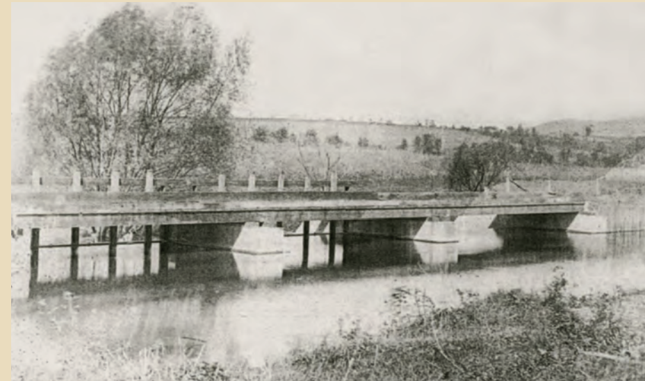
A long bridge carries the canal towpath across the combination overflow-waste weir. The section on the right acted as an overflow allowing excess water to spill back into Lopatcong Creek. In the left background are part of the control mechanisms that operated the waste gates during flooding. At approximately 76 feet in length, this waste weir was the largest in Warren County.
