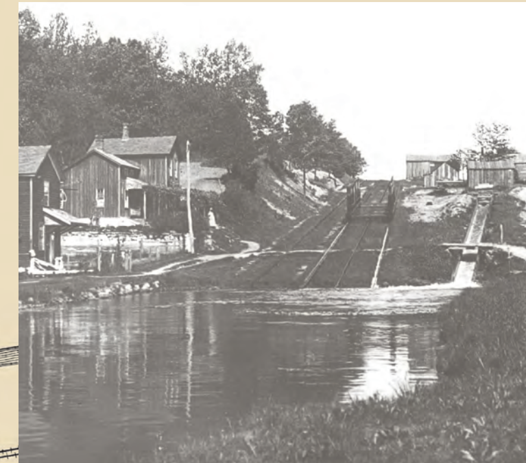
Inclined Plane 6 West and a weigh station are located a short distance to the east, one of only three double tracked planes.
