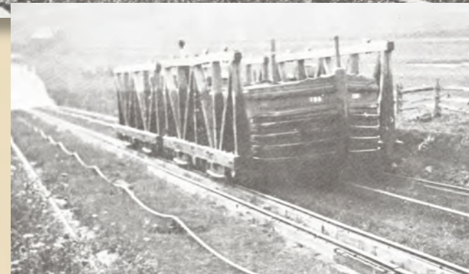
This canal boat was floated into the cradle car at the lower level of the canal and is shown being pulled up the plane. The cradle car rolled on iron rails and was pulled by a cable that looped up and over the plane and back to the powerhouse.
