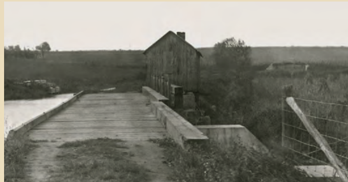
A view looking west down the towpath towards Phillipsburg and across the overflow-waste weir. On the right, in the distance, is the humpback canal bridge over what is now Strykers Road. On the left is a masonry structure where heavy planks could be dropped into a slot acting as a temporary water barrier across the canal prism in case of a break, to drain for maintenance, or to stop navigation at the end of the boating season.
