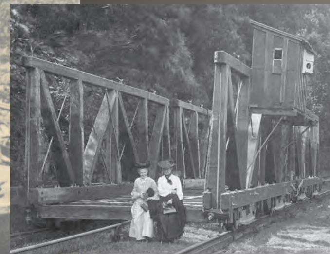
The two ladies sitting on the front of this empty cradle car help to show its massive size. The little shack attached to the car in the upper right was used by the brakeman as he rode up and down the plane with the boats.
