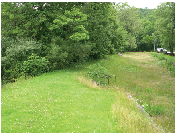
A typical segment of the canal prism's at Saxton Falls remains
