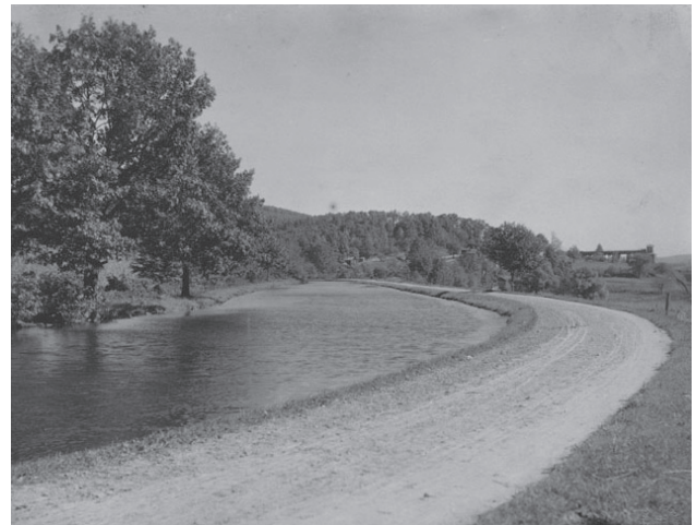
Canal near Port Colden with Plane 6 West in background Photo courtesy of NJ State Archives
